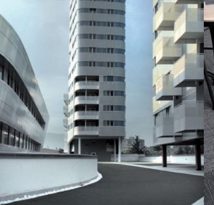
Complesso Futura (Bs)
