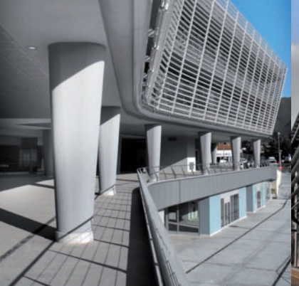
Complesso Futura (Bs)
